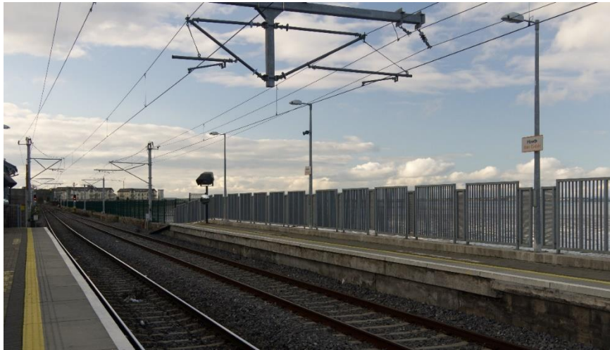
Figure 6-6: Existing head span at Howth Station
