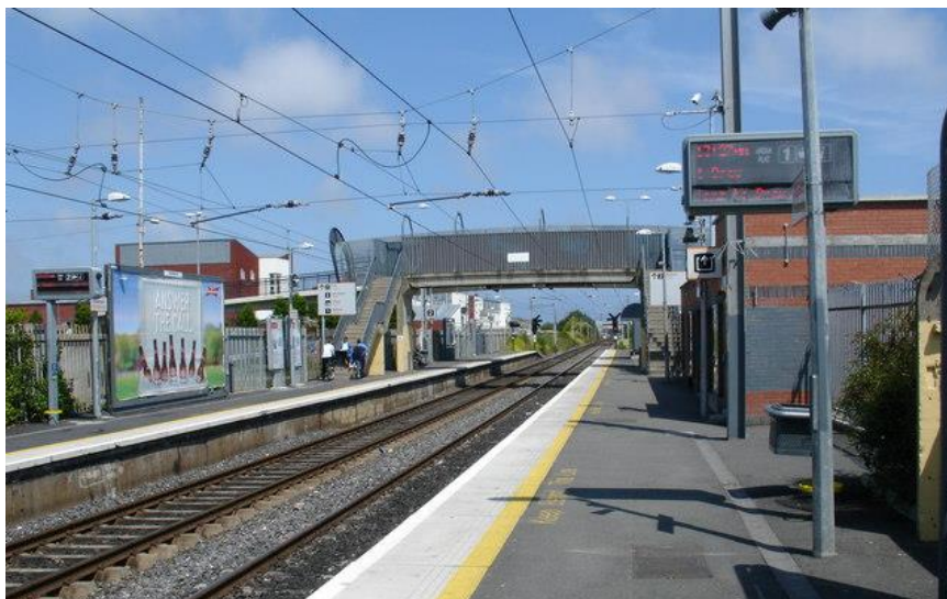
Figure 6-5: Current two track cantilever at Kilbarrack Station
